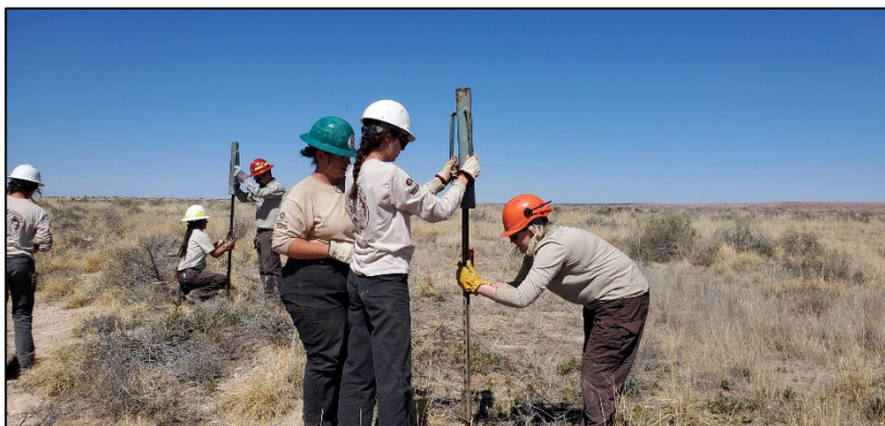
ACE crew and refuge staff work to install new fence.
