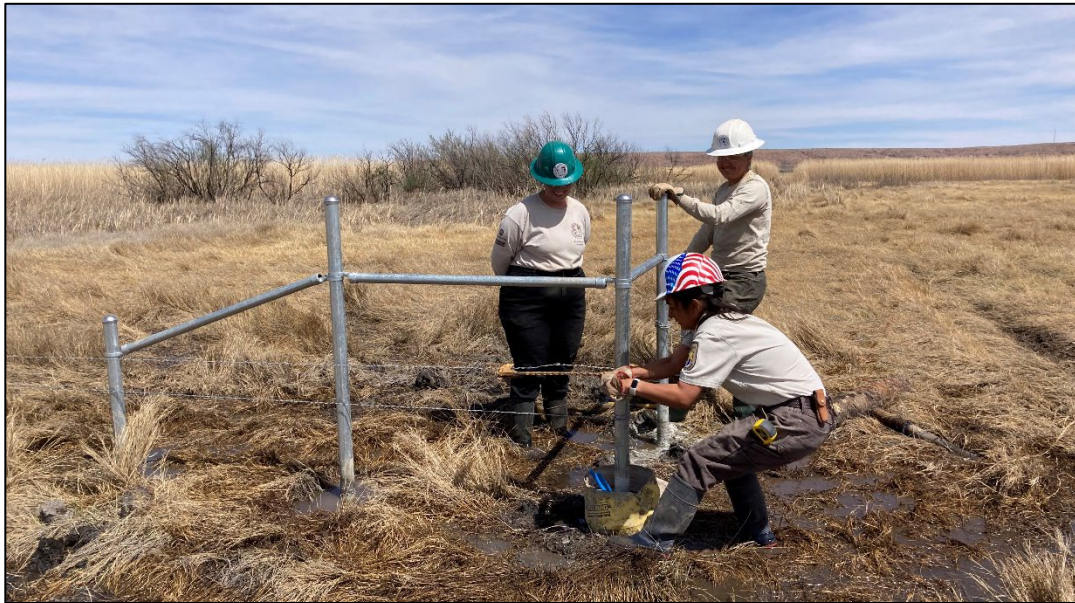
Tightening barbed wire line on a corner brace in Hunter Marsh.
